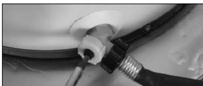
Figure 39 - Draining the water heater.
