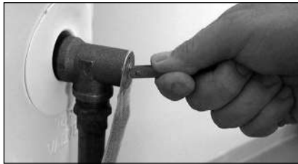
Figure 42 - T&P Relief Valve.
