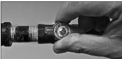
Figure 31 - Gas valve in "on" position
