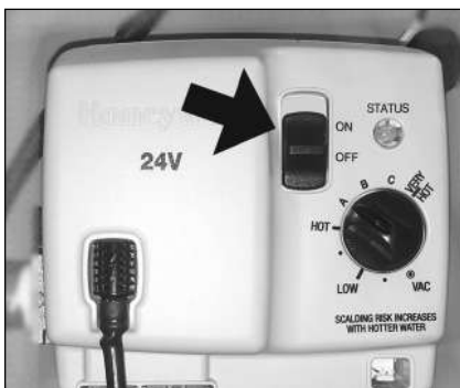
Figure 37 - Turn gas control/temperature knob OFF.
