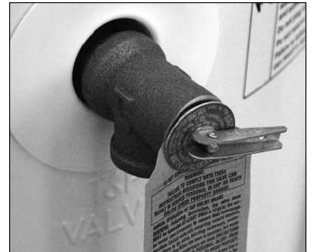
Figure 24 - Temperature and Pressure Relief Valve
