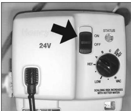
Figure 44 - Turn the gas control valve off.
