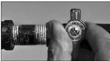
Figure 45 - Gas valve in "off" position.
