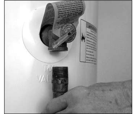
Figure 21 - Removing the T&P Relief Valve discharge pipe.
