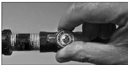
Figure 49 - Gas valve in “on” position.
