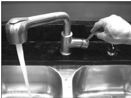
Figure 18 - Let the hot water run until it is cool.
