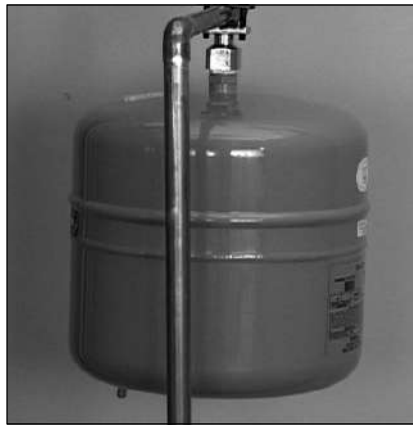
Figure 28 - The Thermal Expansion Tank should be pressurized with air, using a hand pump, to match the home's incoming water pressure.
