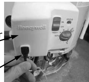
Spark igniter/flame sensor wire
