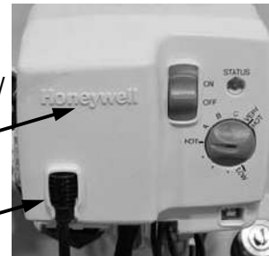
Spark igniter/flame sensor wire
